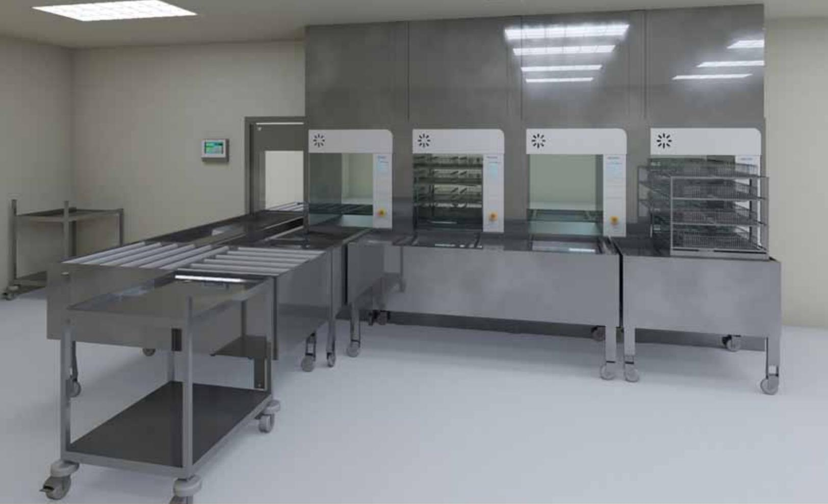
*Automation helps streamline the decontamination process and increase productivity. Operating staff are able to prepare several racks at once and time is saved as loading and unloading of the washers is carried out automatically, without personnel involvement.*
